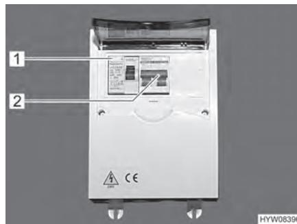
Fig. 116 230 V fuse box with safety cut-out and FI-switch
