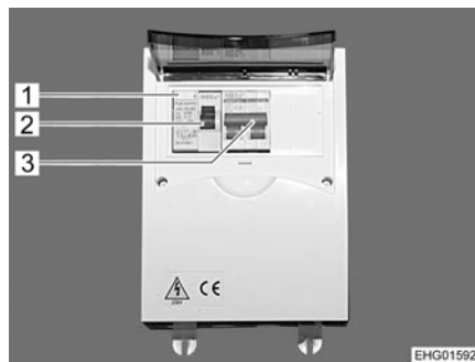
Fig. 171 230 V fuse box with safety cut-out and RCD (main switch)
