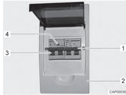
Fig. 56 Safety cut-out and FI-switch (230 V fuse box)
