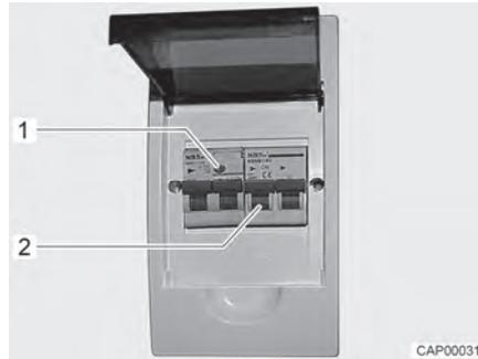
Fig. 90 230 V fuse box with safety cut-out and FI-switch
