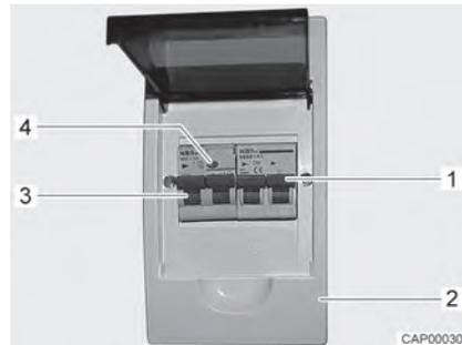
Fig. 78 Safety cut-out and FI-switch (230 V fuse box)
