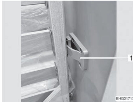
Fig. 61 Locking device (bathroom unit wall)
