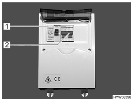
Fig. 79 240 V fuse box with safety cut-out and FI-switch
